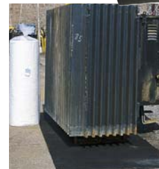
Ideal underneath leaking transformers.
